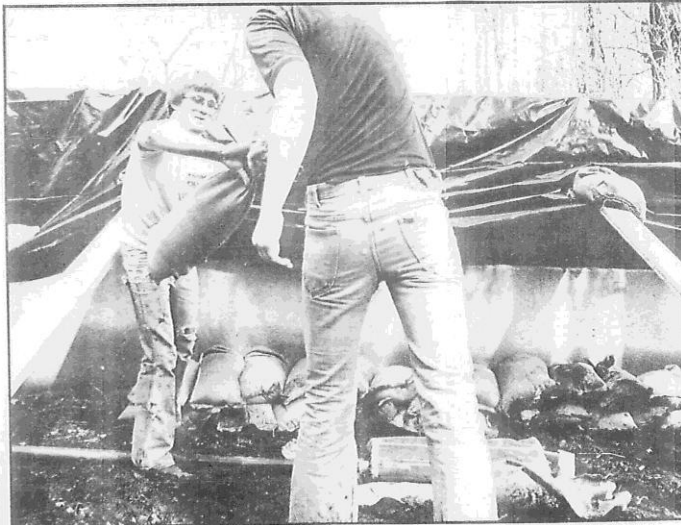
The AGRs try to build the wall of sandbags up high enough to hold back the ever rising waters of the Red River.
