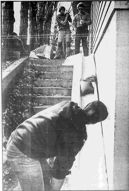
John Peterson and Eric Miller send the sandbags down a slide to a waiting Boyd Zavalney. The slide was used to avoid having to haul the sandbags down the stairs.
